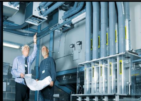
Pneumatic Tubes System
