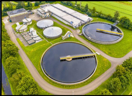
Water Treatment Plant
