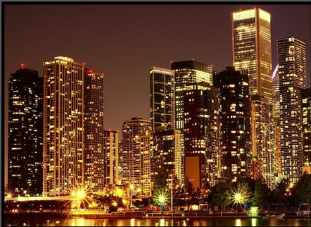
BMS (Building Management System)
